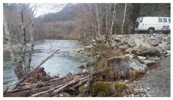
**Figure 5**. Example of rip rap that has been placed in the Middle Fork Snoqualmie River to protect the Middle Fork Road. Photo by Chad Hermandorfer.
