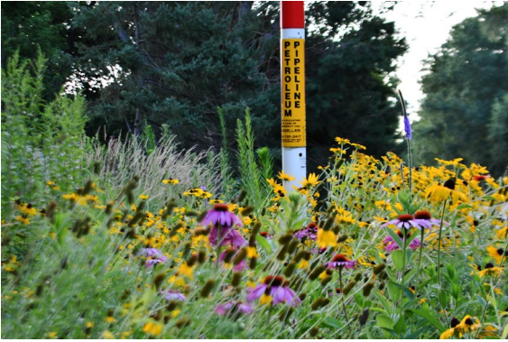
Pollinator habitat blooming along a petroleum pipeline. Photo by Mara Koenig/USFWS.
