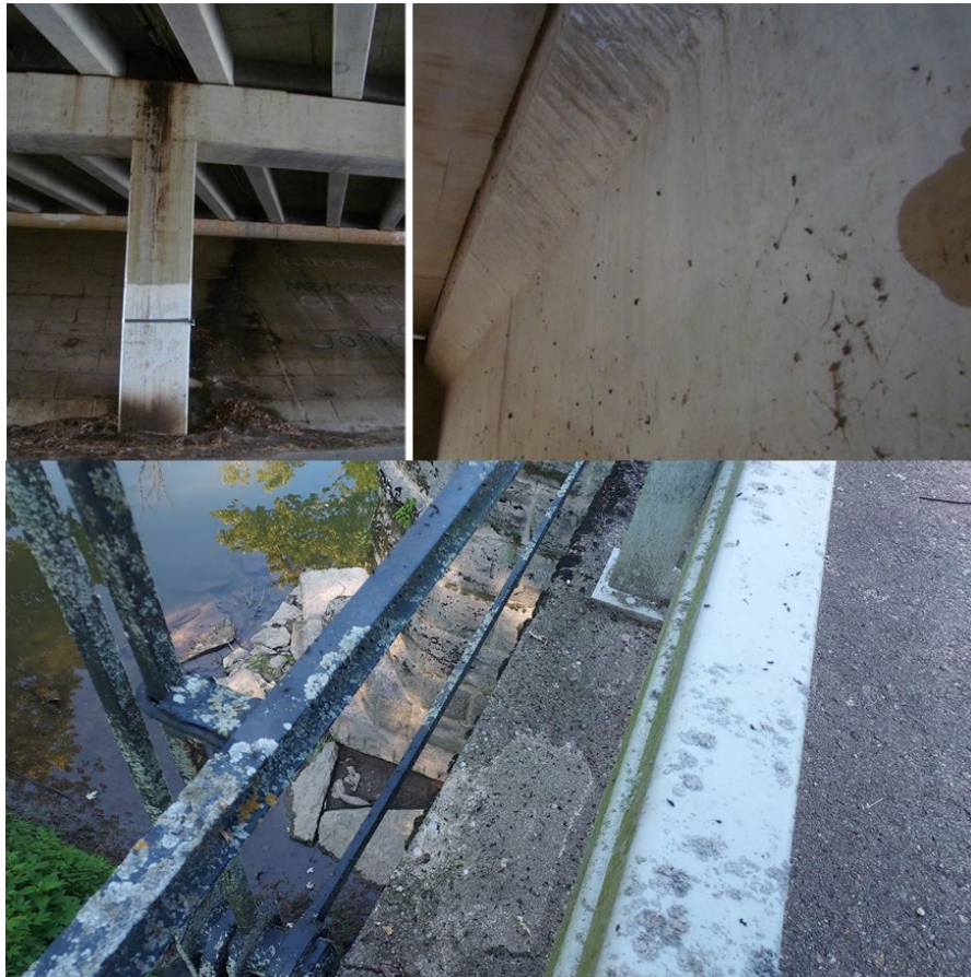
Figure 7. Examples of guano accumulations on bridges. (photos provided by Georgia Department of Natural Resources (top) and Indiana Department of Transportation (bottom)).
