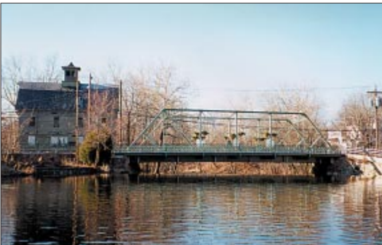
Iron truss bridge, Borough of Bloomsbury
