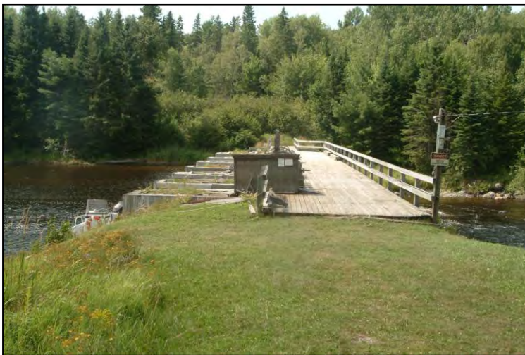
(Left) Telos Dam (2010 Photo)
