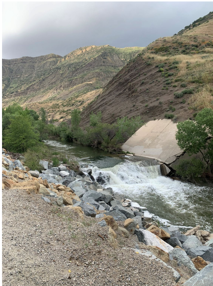
USGS nonfunctioning gauging station and weir
