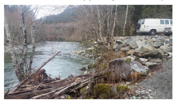
Figure 26 - Example of rip rap that has been placed in the MF to protect the Middle Fork Road.
