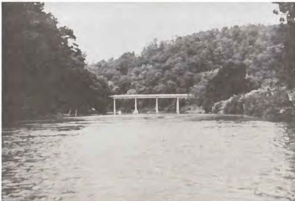
Figure II-1 - U.S. Highway 221 crosses the New River within the study area.
