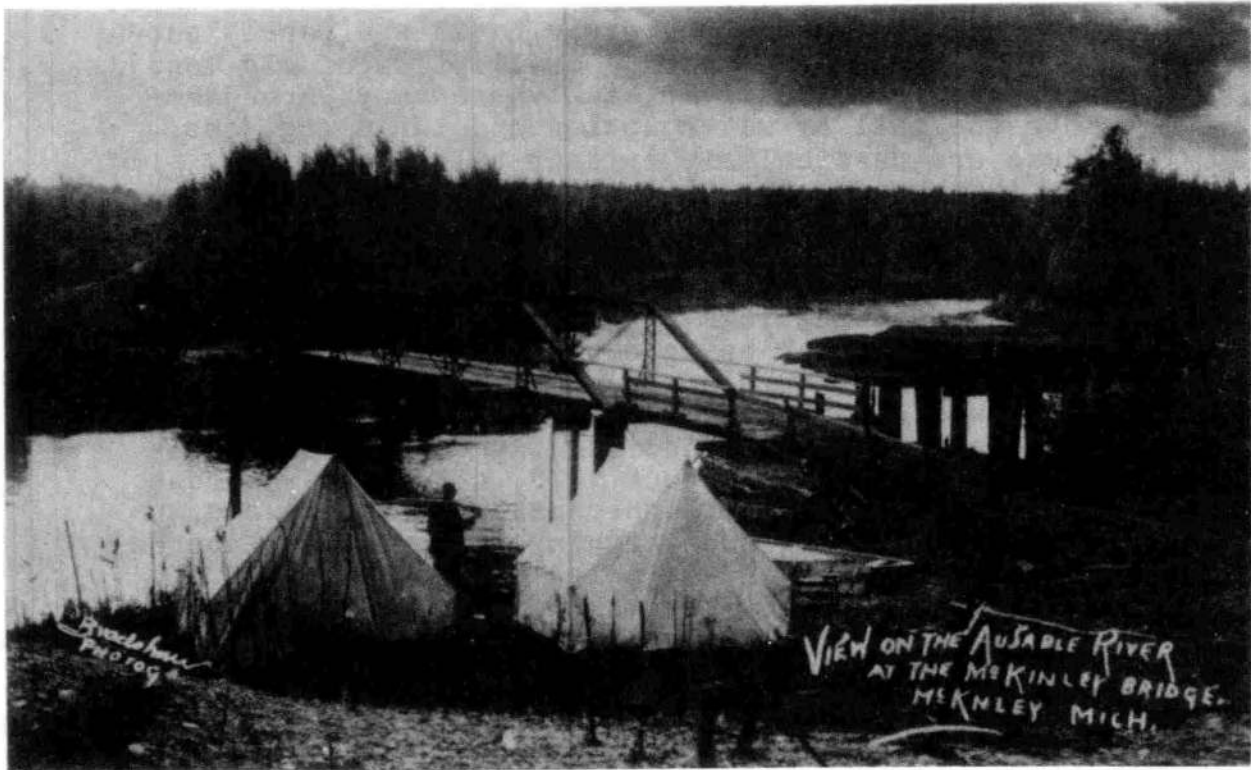
McKinley Bridge during the late 1800's . Courtesy - Michigan History Division
