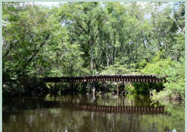
Relict Bridge over Black Water Creek
