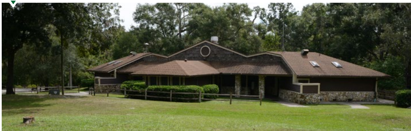
Concessions Building at Kelly Park
