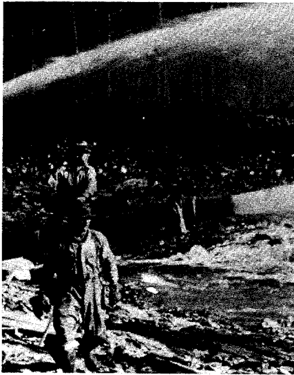
Hydraulic monotors on the Ore Grande Mine in the 1930's.
