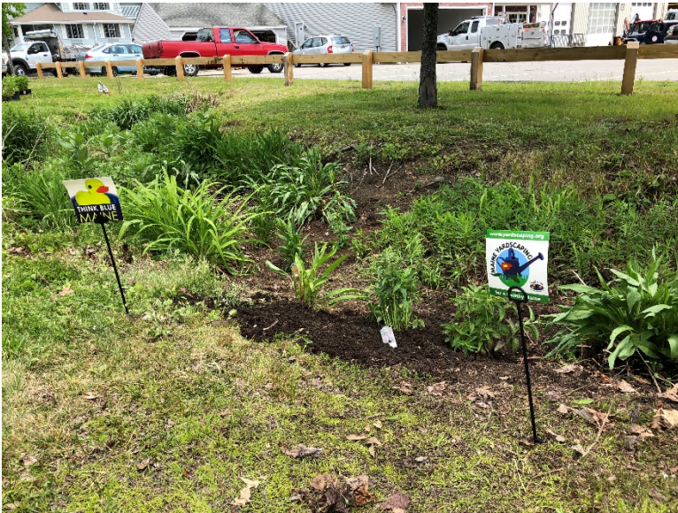
Native plants in this new biofilter outside Kittery Town Hall will help treat stormwater runoff. Photo: Kristie Rabasca
