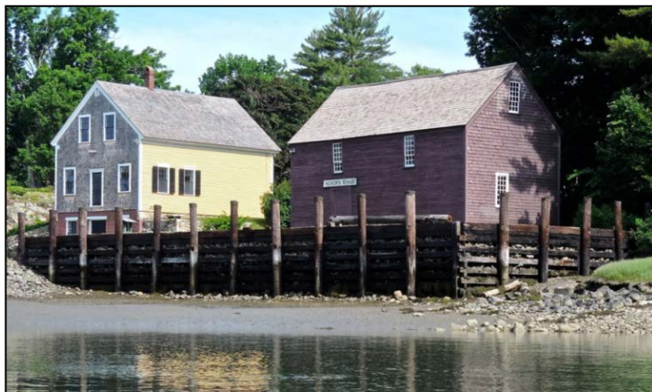
John Hancock Warehouse (right), a National Register site, and George Marshall Store Gallery (left). Both sites are owned by Old York Historical Society.
