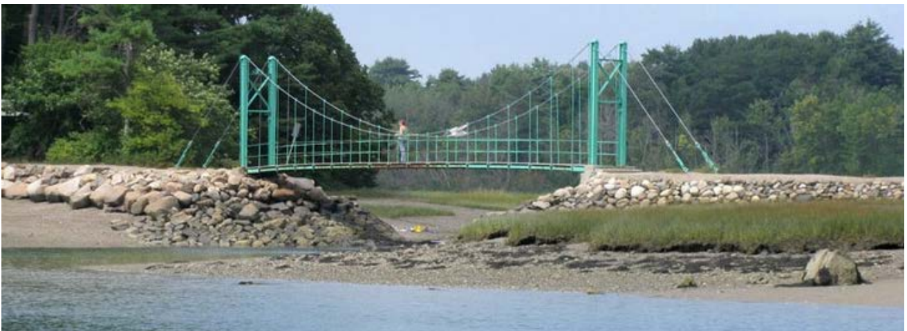
Wiggly Bridge and adjacent pedestrian causeway viewed from the York River.
