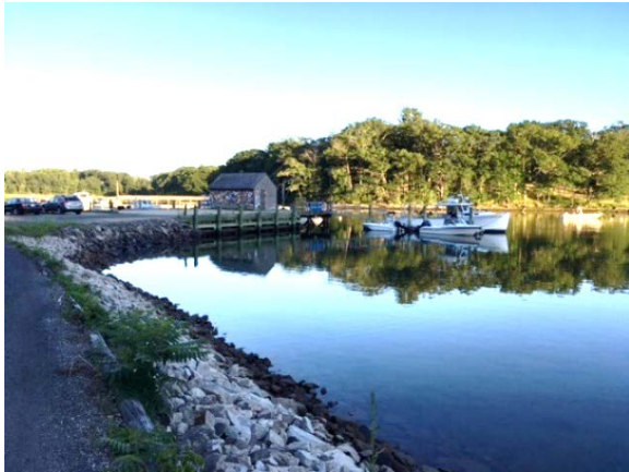
Rip rap along Lindsay Road extending to John Hancock Wharf. Photo: Joan LeBlanc
