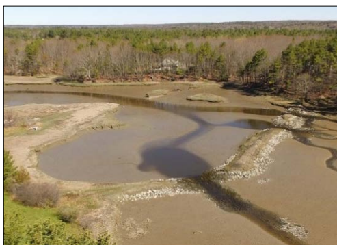
Remains of tidal mill dam on Dolly Gordon Creek (left and center). This dam was first constructed by 1705 by John Pickering and is slightly downriver from the site of the 1634 mill, which is believed to be the earliest tidal mill site in the English colonies. Remnants of dam and mill site of former Bartlett-Briggs grist mill on York River (right). Photos: Emerson Baker (left), Stefan Claesson (center), and Northeast Archaeology Research Center (right)
